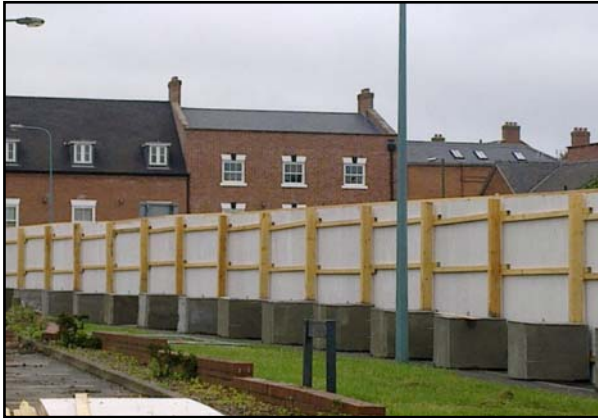
Figure 8 - Typical kentledge block hoarding
