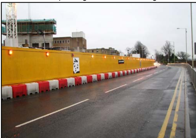
Figure 3 - Typical hoarding with vehicle barrier
