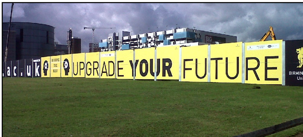
Figure 10 - Typical Proprietary Hoarding with Advertising Panels
