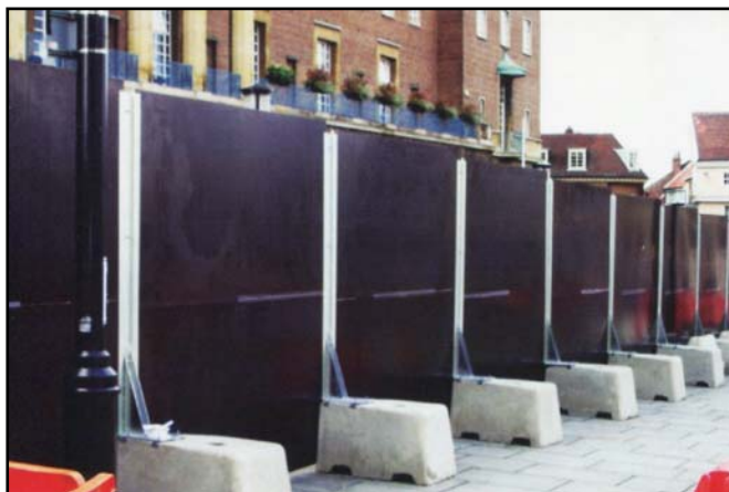
Figure 7 - Typical proprietary hoarding with foundation blocks
