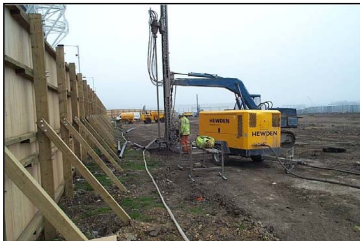
Figure 1 - Typical site hoarding – site view
