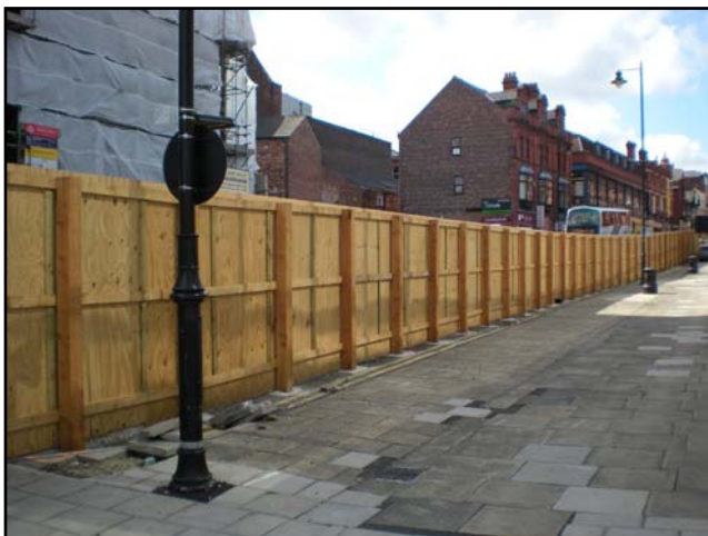
Figure 6 - Typical timber post-in-hole hoarding
