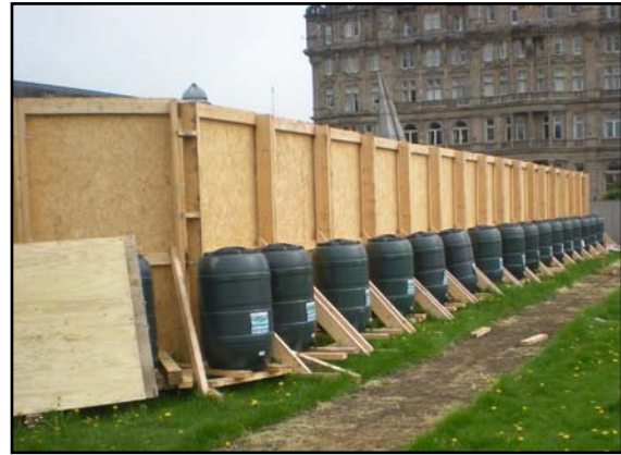
Figure 9 - Typical ballasted hoarding
